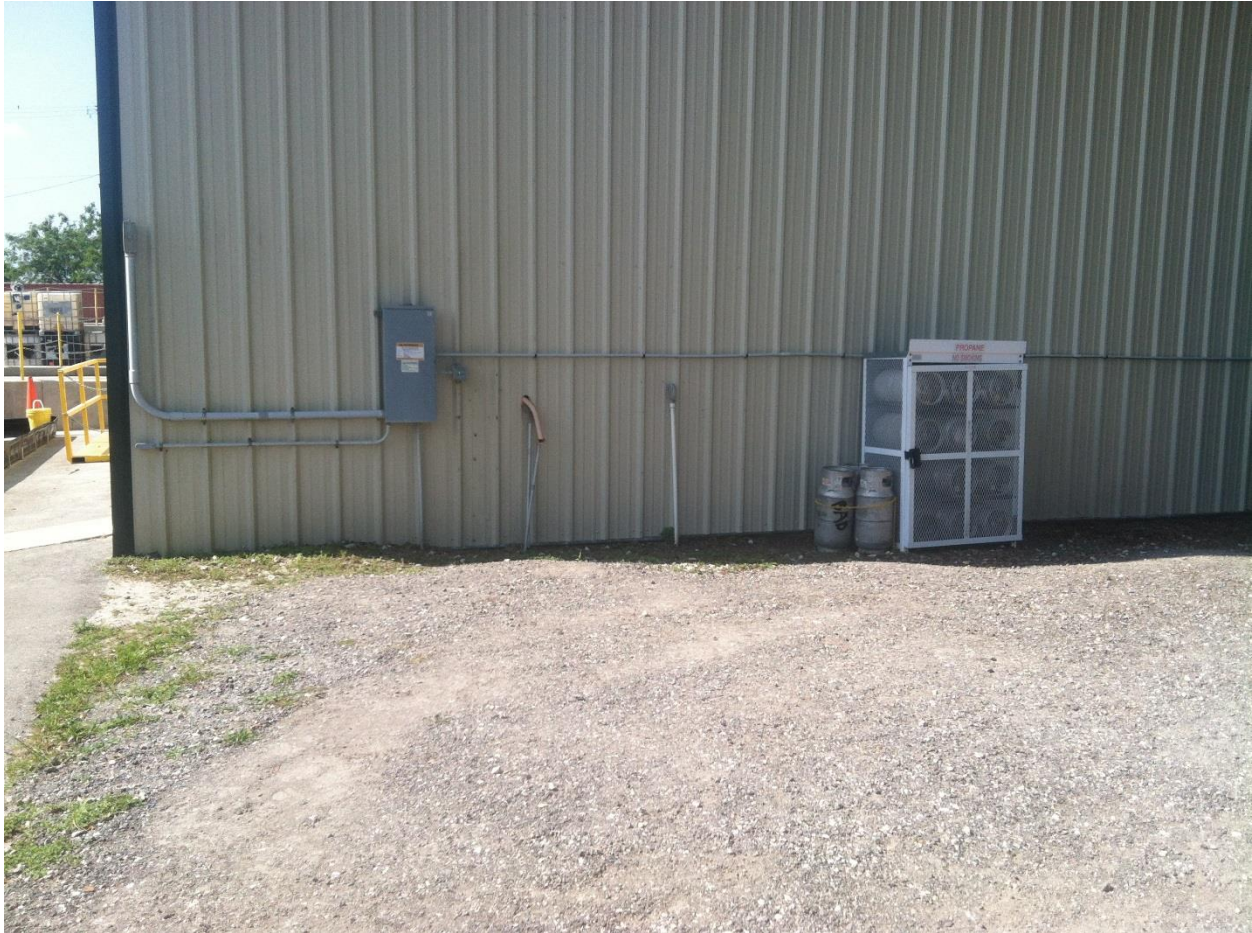
SWMU 19 – Proposed location of the Oil-Water Separator. This photograph shows the proposed location of the Oil-Water Separator, facing south. The unit was never installed. Photo taken 2016.
