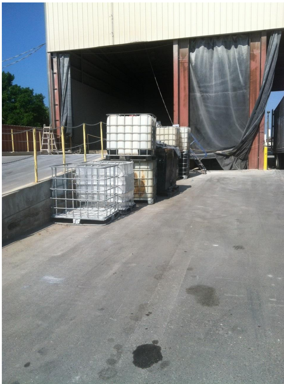
SWMU 20c – Location of the Bulk Container Storage Area (BCSA). This photograph shows the proposed location of the Bulk Container Storage Area, facing west. Photo taken 2016.
