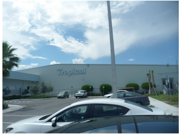
Tropical Shipping New Warehouse
