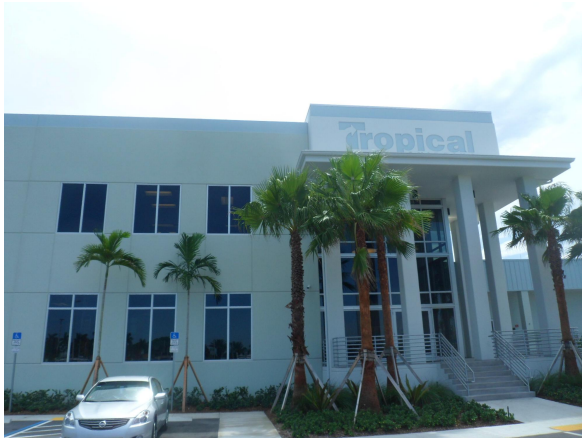
Tropical Shipping New main office
