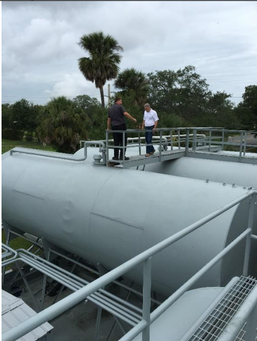
Photograph 7 – SPCC Inspection June 7, 2017, of recently painted horizontal ASTs #3 and #2.
