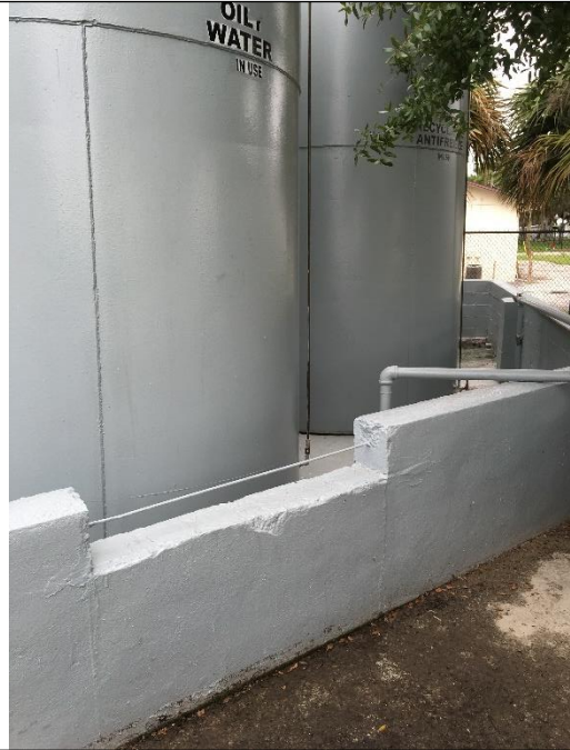
Photograph 10 – View north of containment wall between AST #5 and #6 (not shown) and ASTs #7 and #8 (shown).
