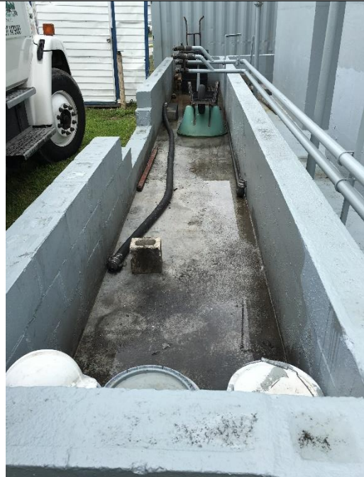
Photograph 12 – View west of containment overflow area for pipes used to load/unload ASTs #7 and #8 (oily water and recyclable coolant). South containment wall for Area 2 on right.
