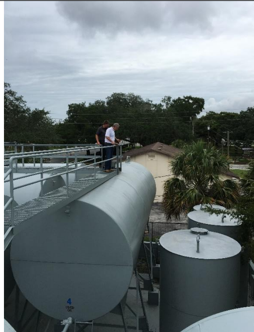
Photograph 8 – SPCC inspection photos showing horizontal AST #4, and vertical ASTs #7, #8, and #9 (view north).
