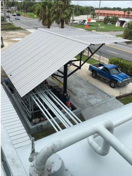
Photograph 11 – Overhead metal canopy covers the active loading containment area where used oil is pumped between oil trucks and ASTs #1-#6. French Avenue (Hwy 17-92) is in background.
