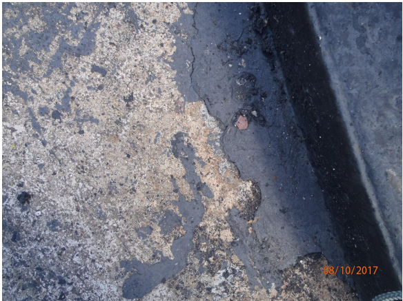
Black coating/sealant wearing off
