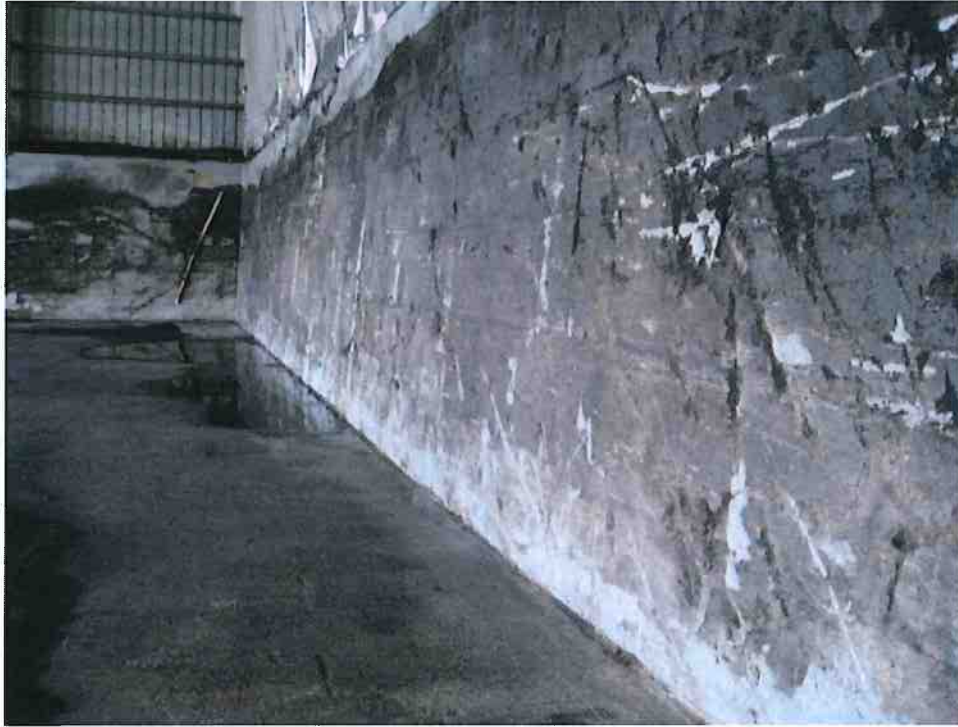
Former Soils Treatment Storage Building Walls after Pressure Washing
