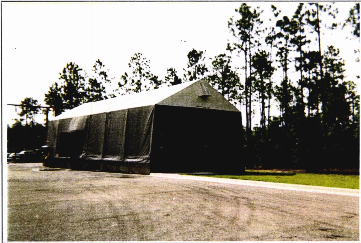
Photograph 3: Tank farm (view to the southeast)
