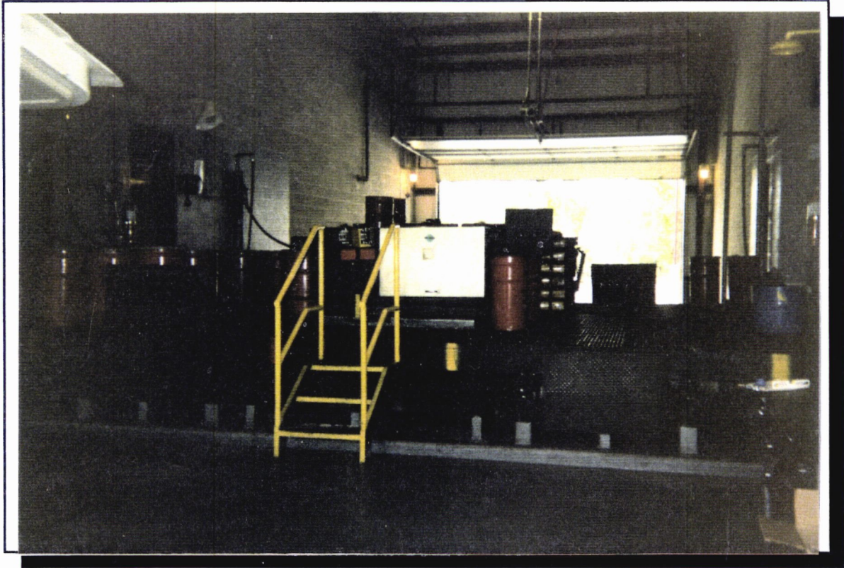
Photograph 5: Return/fill shelter (view to the south)
