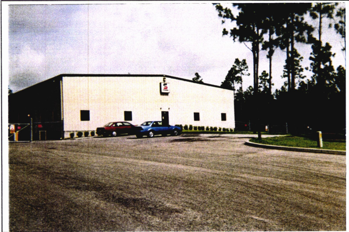
Photograph 1: Facility entrance (view to the west)
