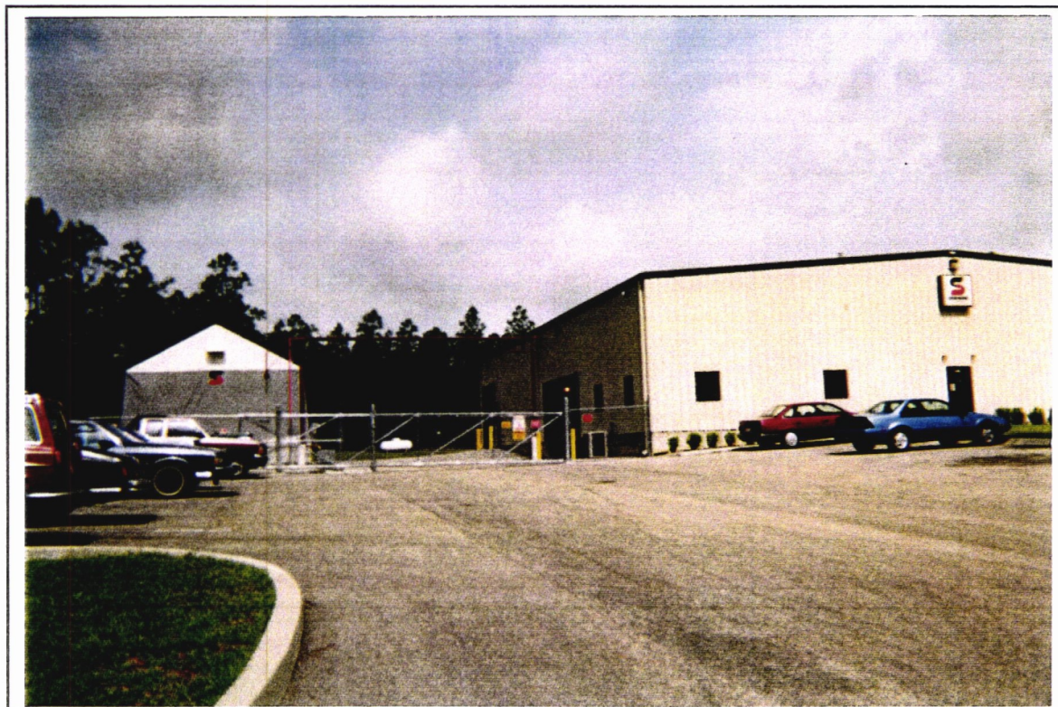
Photograph 2: Facility entrance and tank farm (view to the west)
