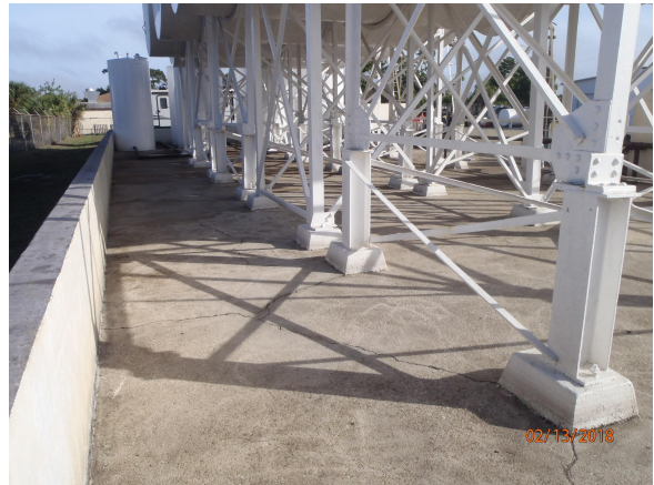
Photo 8 - cracks in containment floor
