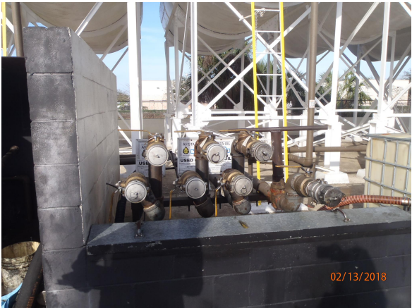
Photo 1 - tank fill/drain ports
