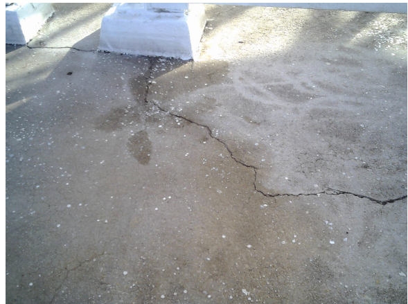
Photo 16 - cracks in containment floor
