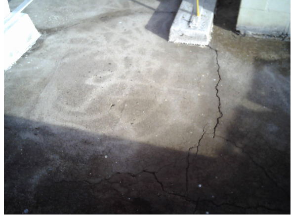
Photo 16 - cracks in containment floor
