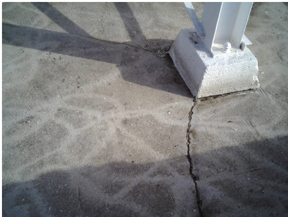
Photo 15 - cracks in containment floor
