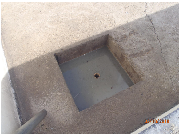
Photo 11 - drain sump
