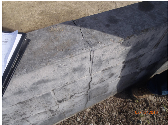
Photo 10 - crack in containment wall
