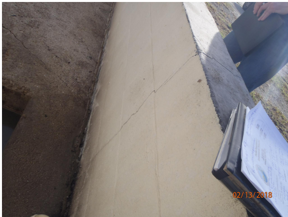
Photo 9 - crack in containment wall
