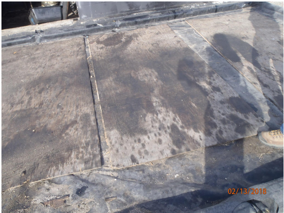
Photo 6 - stained plywood
