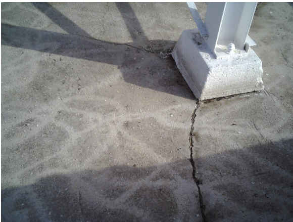
Photo 15 - cracks in containment floor
