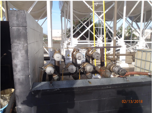
Photo 1 - tank fill/drain ports
