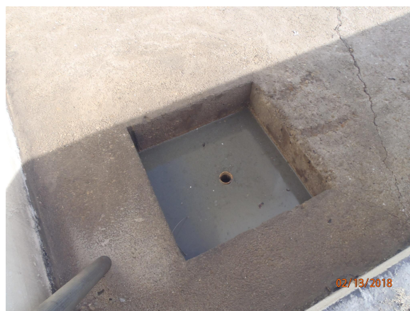
Photo 6 - Drain sump
