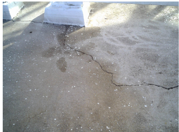
Photo 13 - cracks in containment floor
