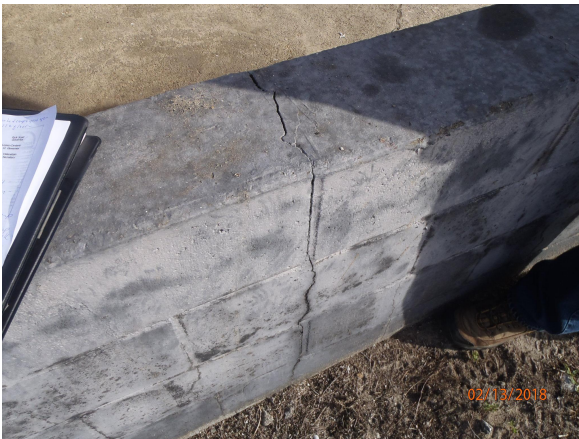
Photo 10 - crack in containment wall
