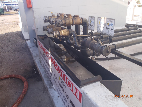
Photo 16 - retrofitted containment
