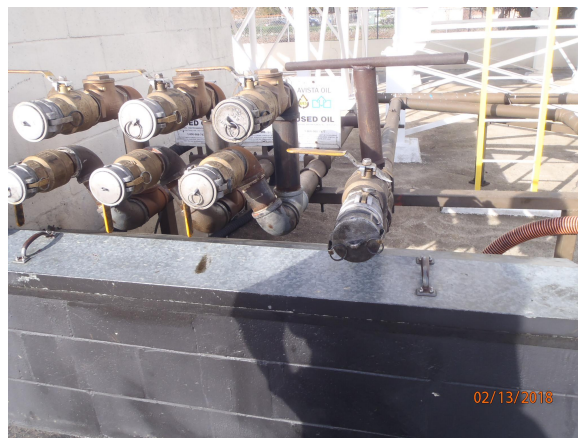
Photo 4 - Drain/fill port valve on right
