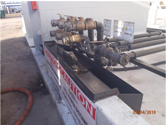
Photo 16 - retrofitted containment
