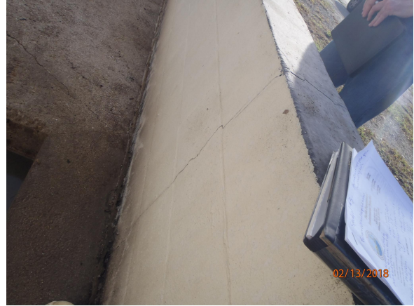
Photo 11 - cracks in containment floor
