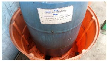
Used oil/stormwater is present in the maintenance shop used oil containment
