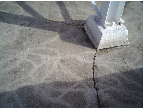
Photo 12 - cracks in containment floor
