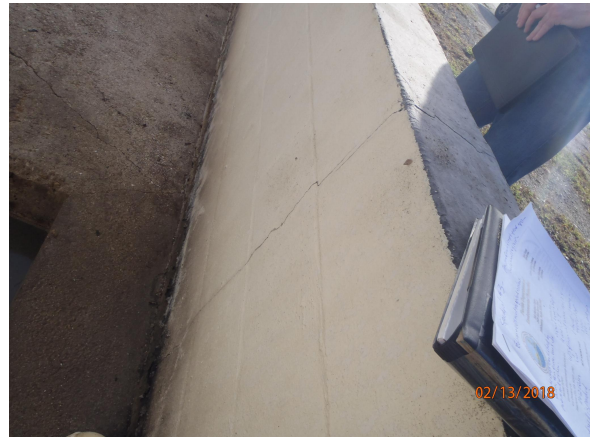
Photo 9 - crack in containment wall
