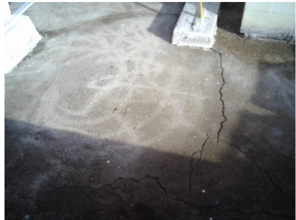
Photo 11 - cracks in containment floor
