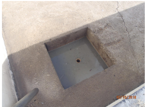
Photo 6 - Drain sump
