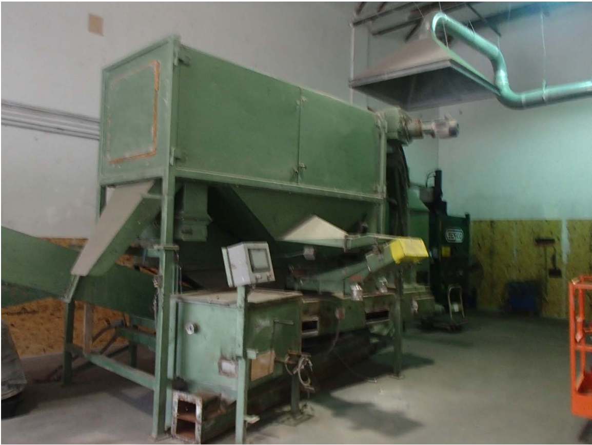
Figure 2. LSS1 processing machine. Ductwork is visible in top right of photograph.
