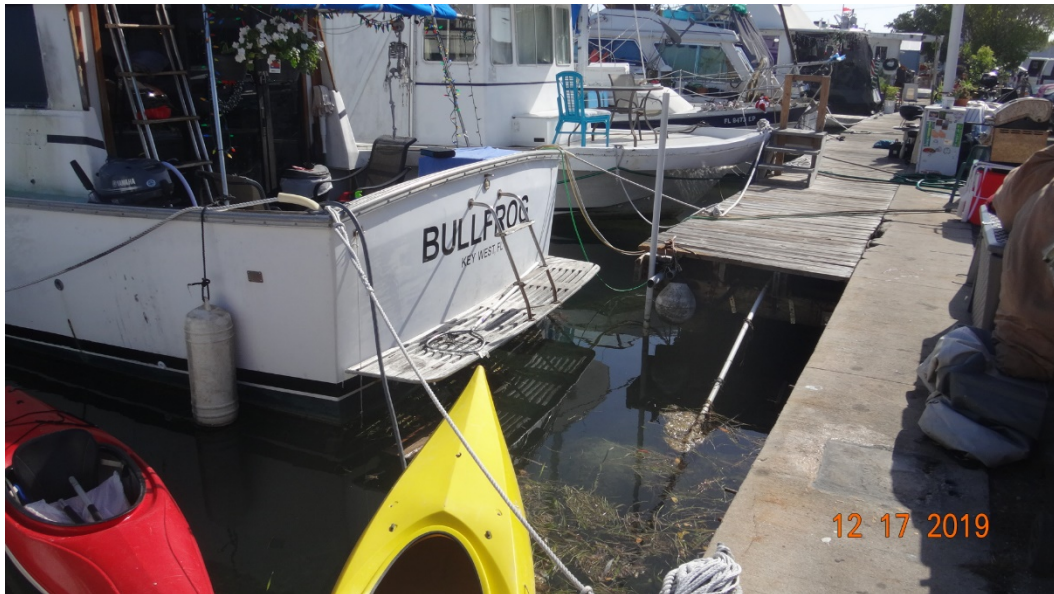
Photo 1: Looking at marginal dock within leased area. Note: Portion of marginal dock is missing.
