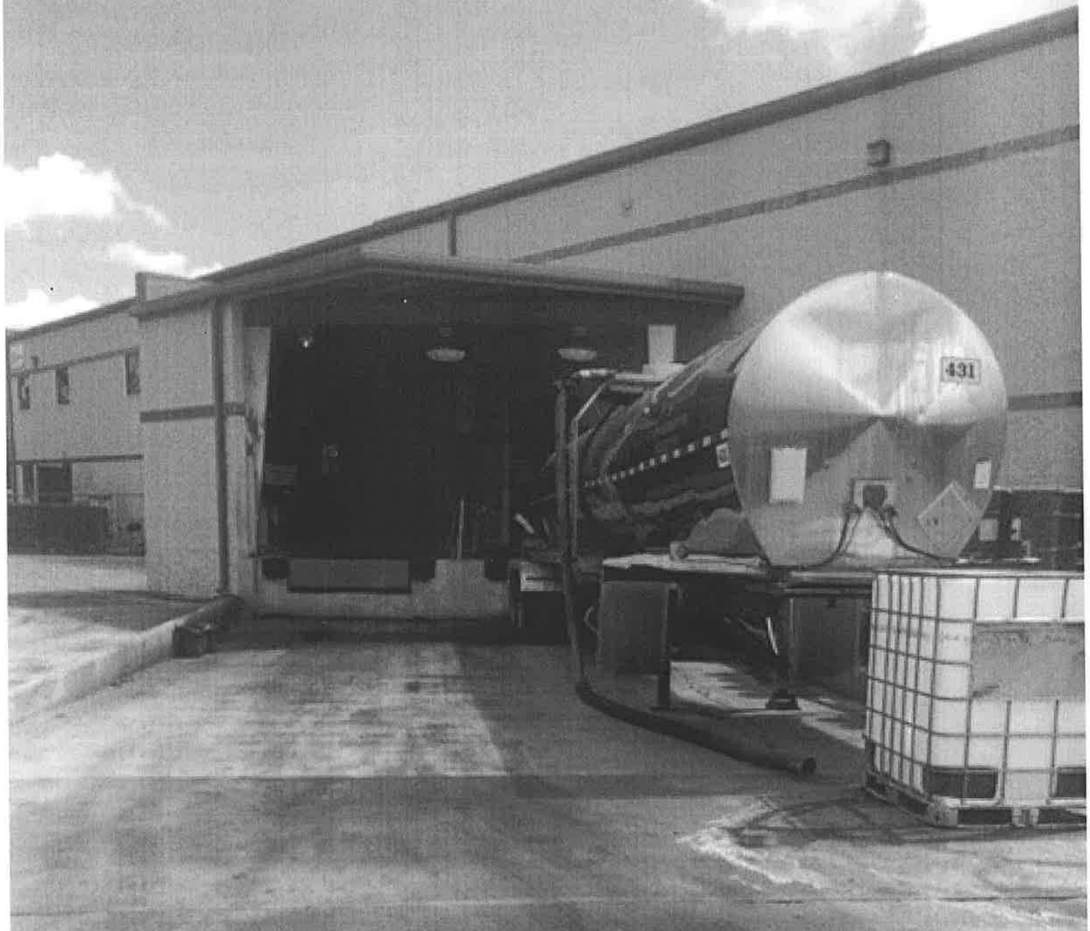
2018 SK Sanford Back Loading Dock/Oily Water Tanker Facing Southeast
