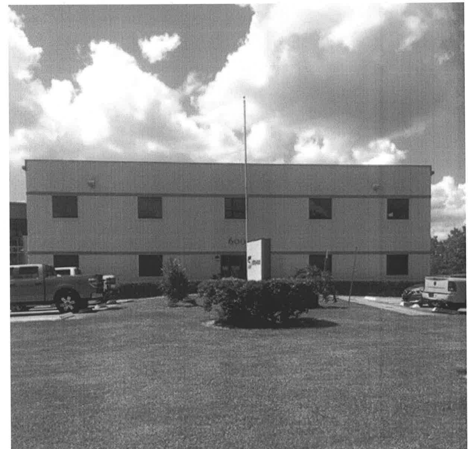
2018 SK Sanford Front Building Facing West
