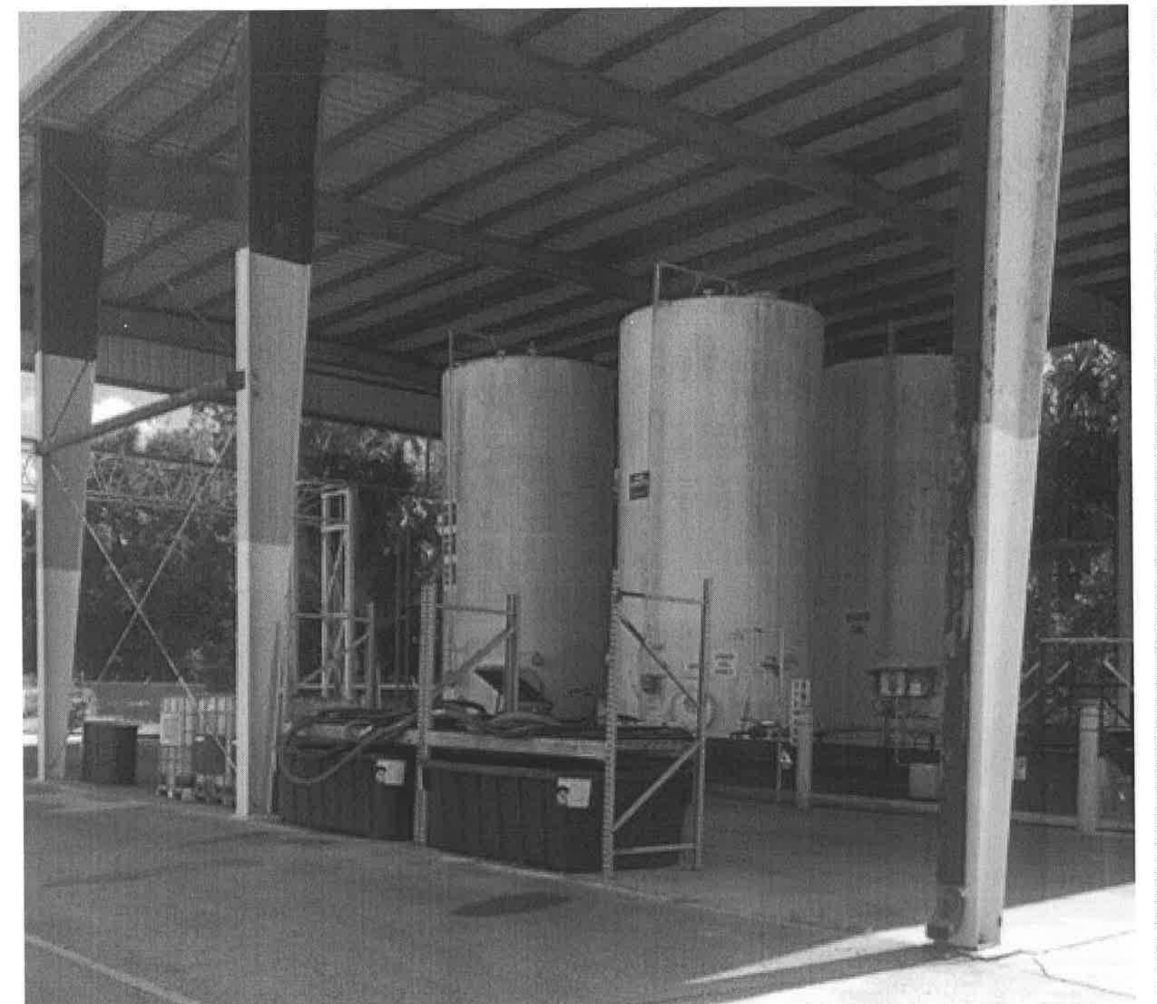
2018 SK Sanford Tank Farm Facing Southeast
