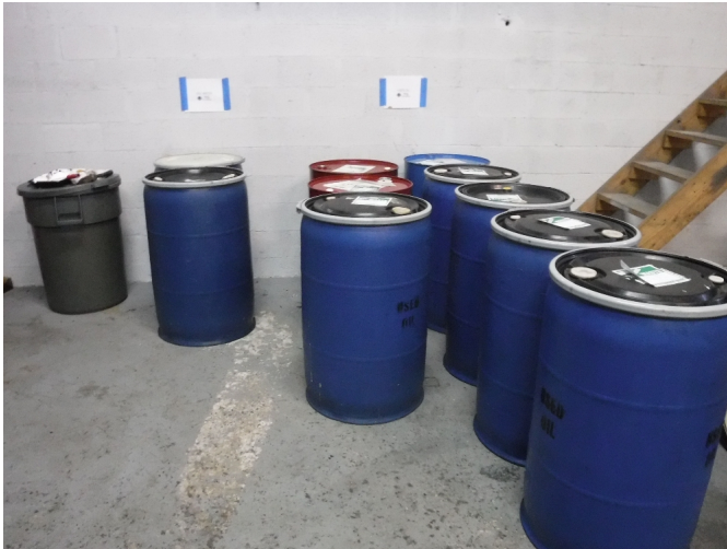
UO drums without secondary containment
