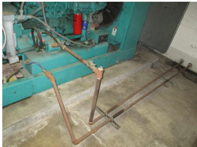
GenSet Aboveground piping connection
