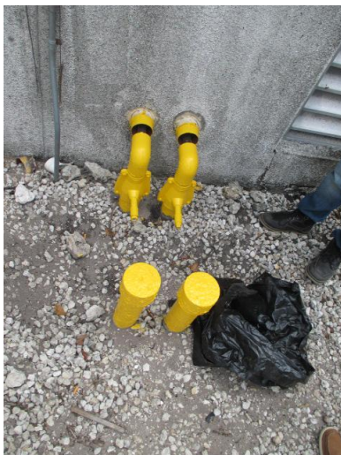
Piping transition into Generator Room
