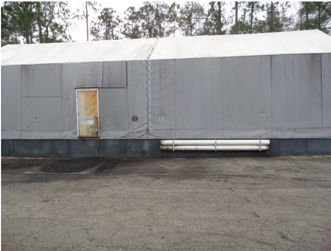
Photo 1: Exterior of the Storage Tank Farm
