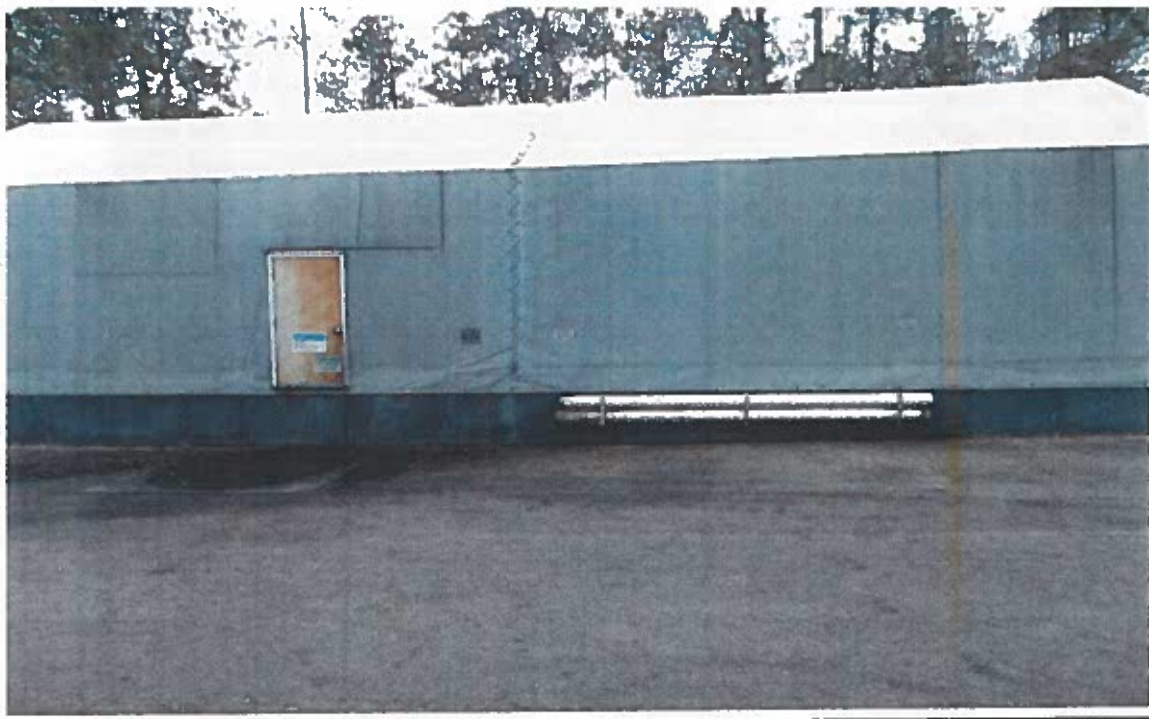
Safety Kleen Systems, Inc. – Tallahassee FL. RCRA Permitted Tank Farm. Observed two 15,000-gallon used oil tanks and one 15,000-gallon RCRA permitted tank (Tank). The tank farm is constructed with a concrete floor four to five-foot high concrete walls and covered by a rigid canvas material. Photograph 1 taken at 12:22 p.m. WK.
