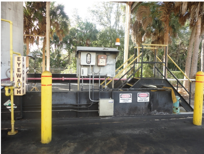
3. Tank farm release detection and signage
