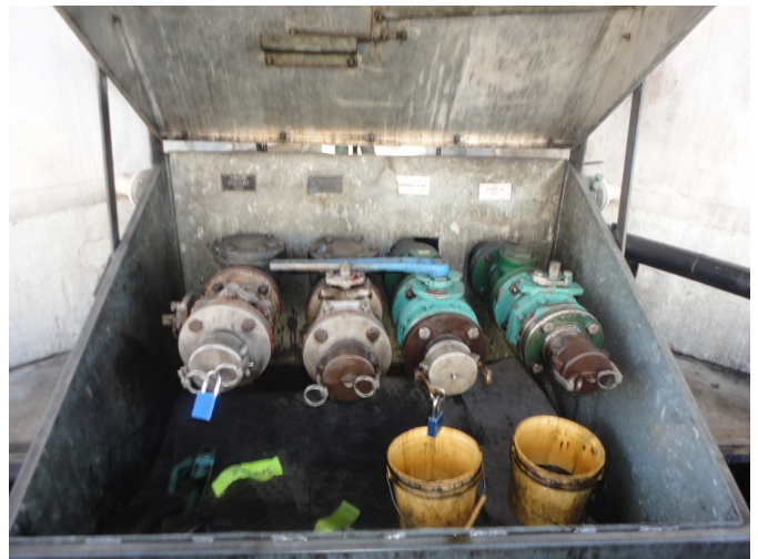
4. Tank spill bucket and fill ports
