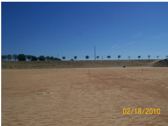
Limits of Waste Marker top of Berm
