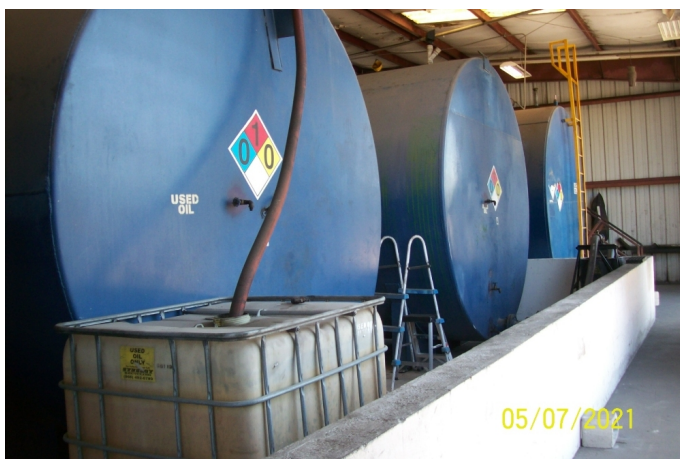
Used oil tanks in secondary containment
