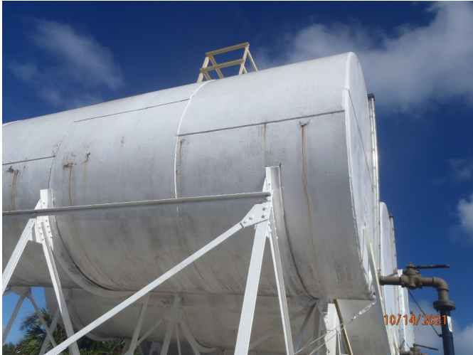
containment structure drain port/valve
