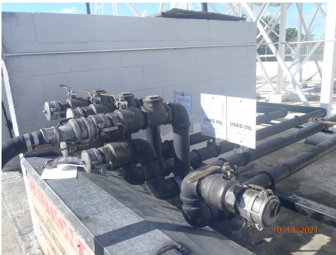
storage tank ports
