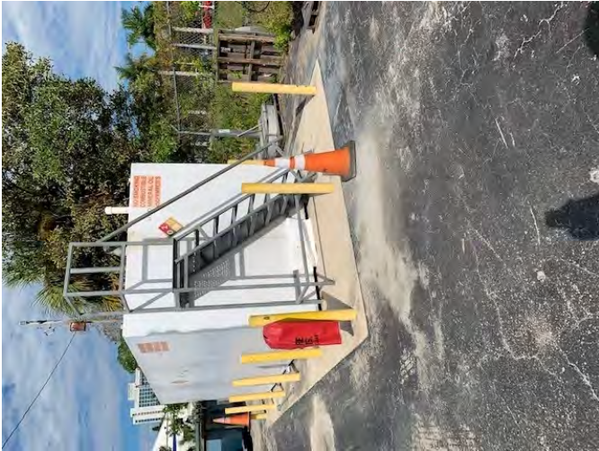
used oil storage tank
