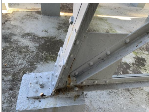
Photo #11: Concrete footing of AST #4, showing minor rust. Painted last in 2016-17.
