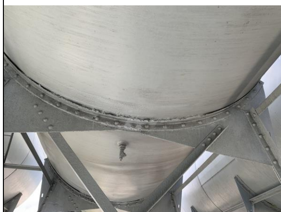
Photo #9: View of the underside and support cradle for AST #2.
