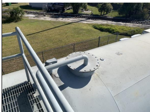
Photo #5: View of AST #5 with inlet pipe and vent. Facing southeast across neighboring property and RR tracks.
