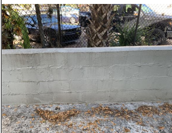
Photo #10: View of sealed concrete wall which is part of Secondary Containment Area 1. Facing north.
