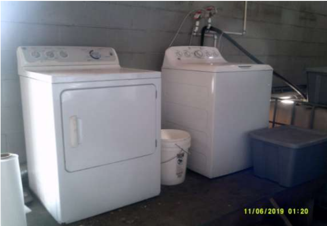
P-2 WASHER & DRYER INSTALLED AT RAG RECYCLING FACILITY SUPPLY
