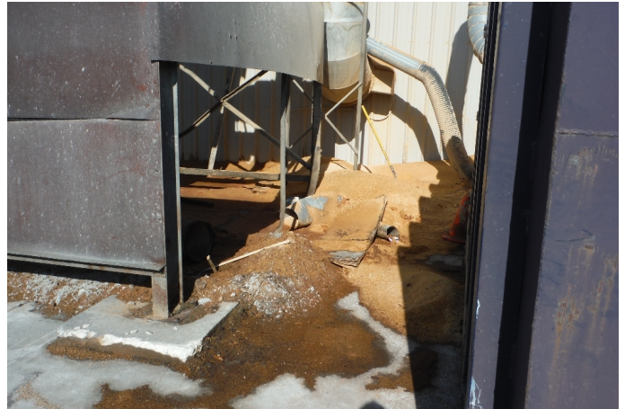
Photo 4 - Baghouse dust on concrete pad
