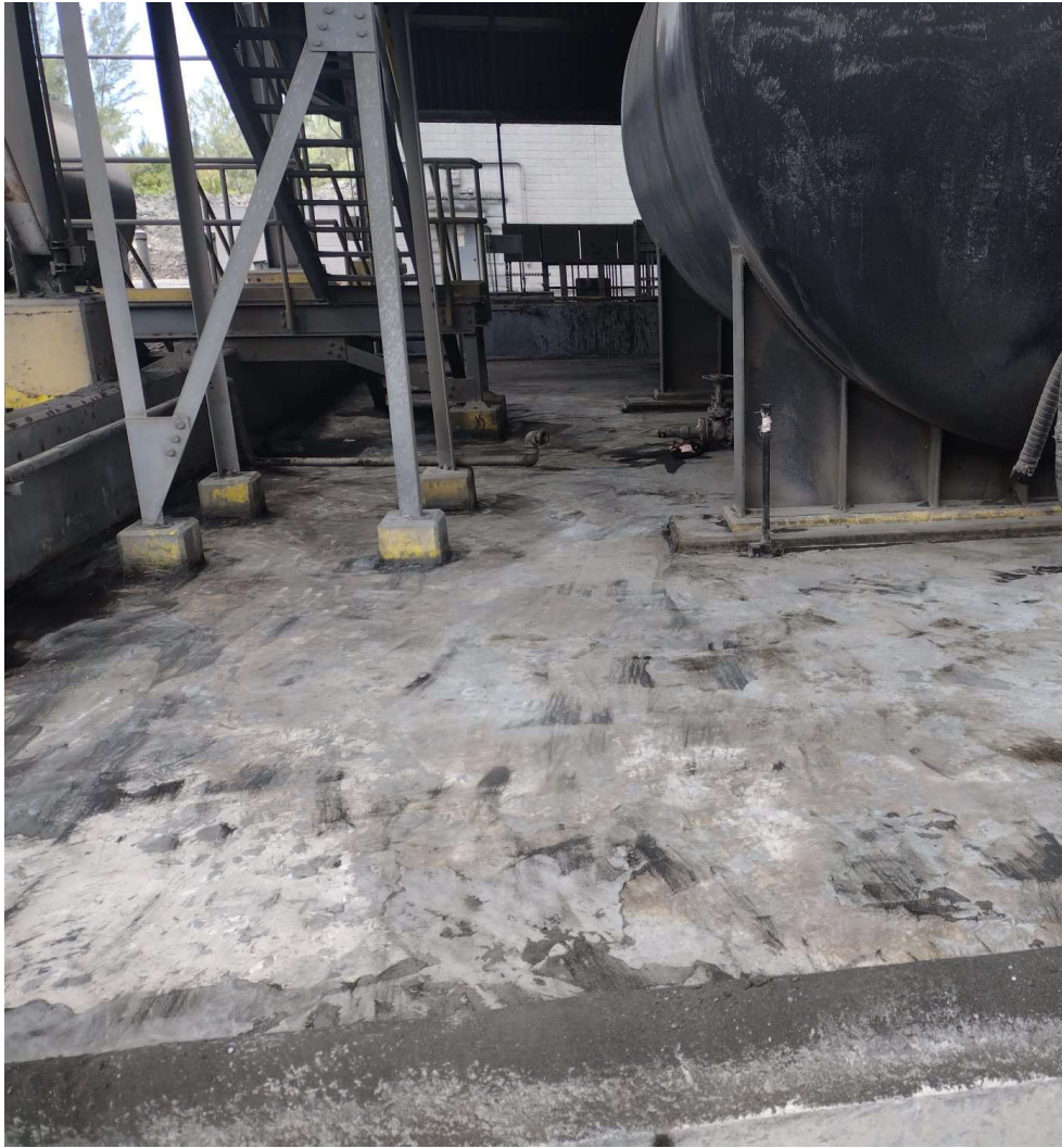
Item 6 Corrected – Containment area of used-oil day tank cleared of material buildup
