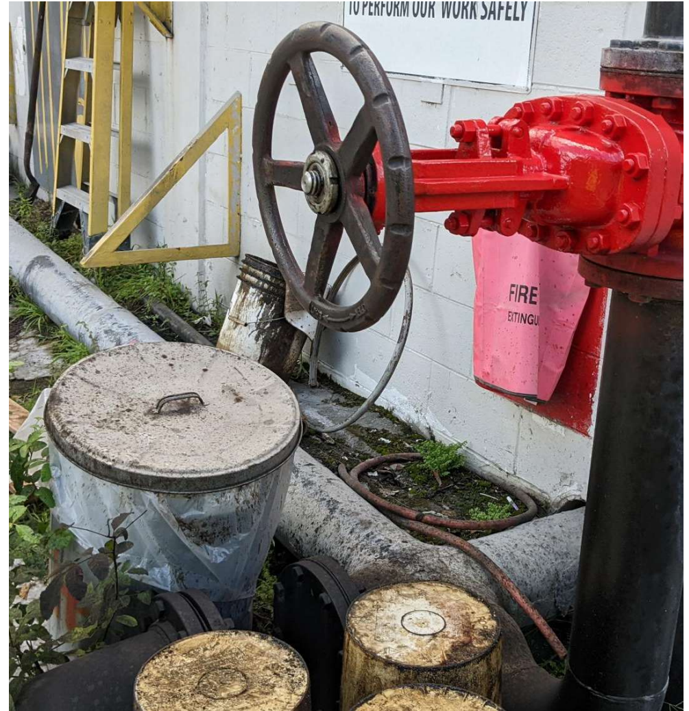
Item 8 Corrected – Leaking valves and connection points repaired at Used Oil Receiving.
