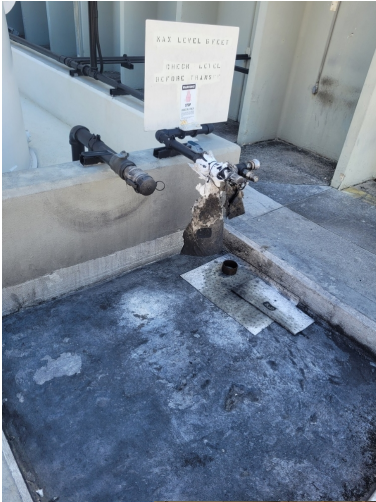
Connection Pipes at the Used Oil Tank Area
