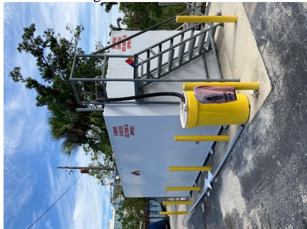
Used oil storage tank
