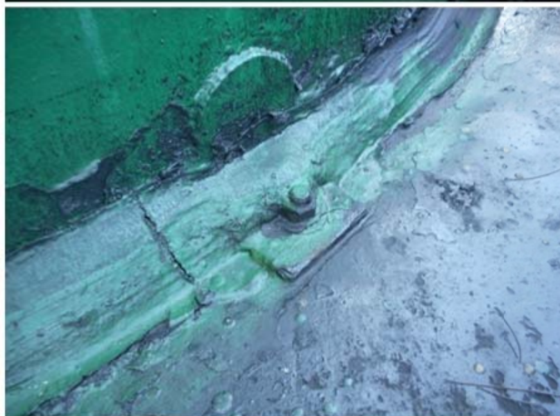
TANK ANCHOR & BPE COVERED WITH FIBERGLASS
