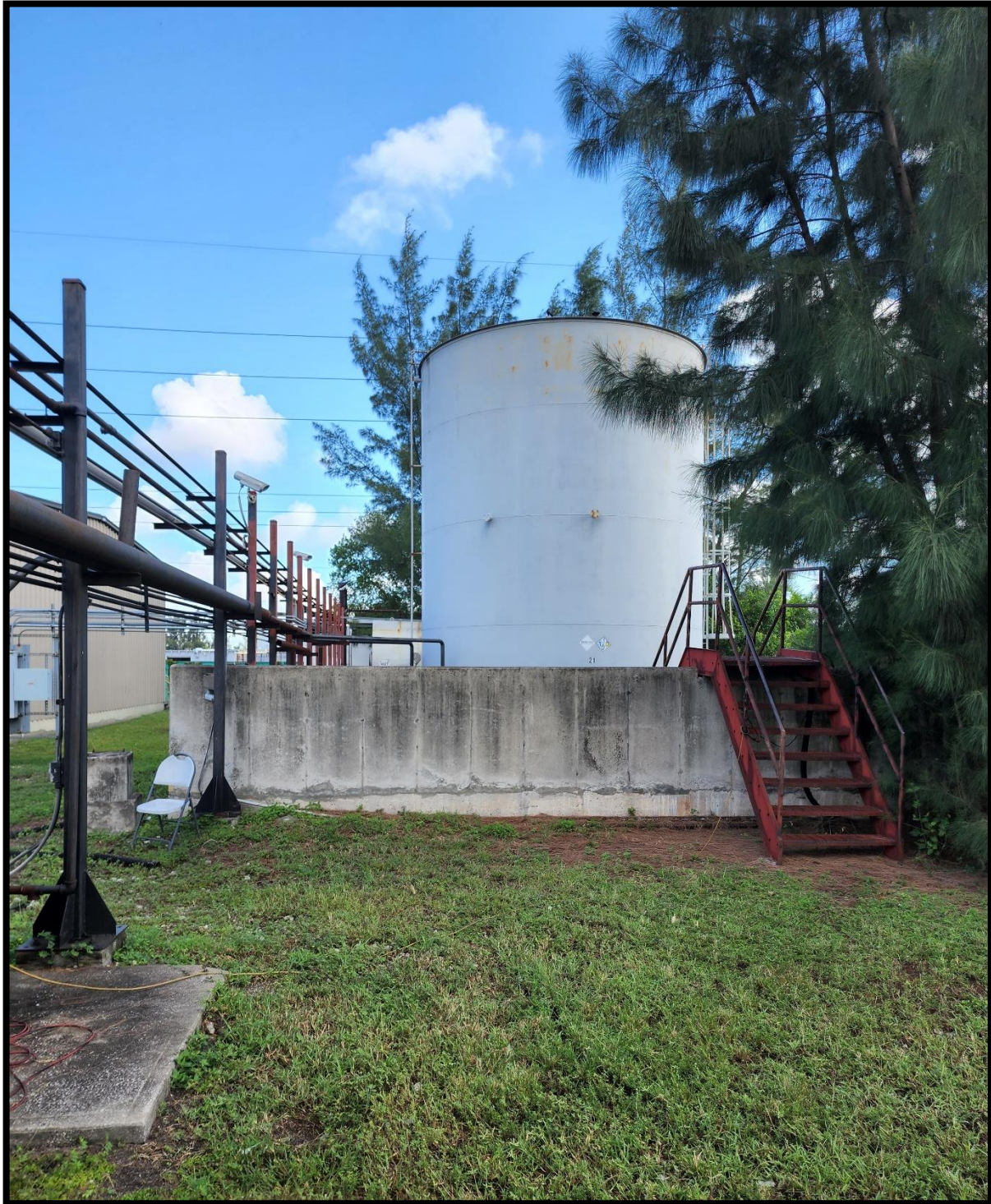
Photo 10: Tank 21 and Tank 22 in Secondary Containment #4 (View from the South)
