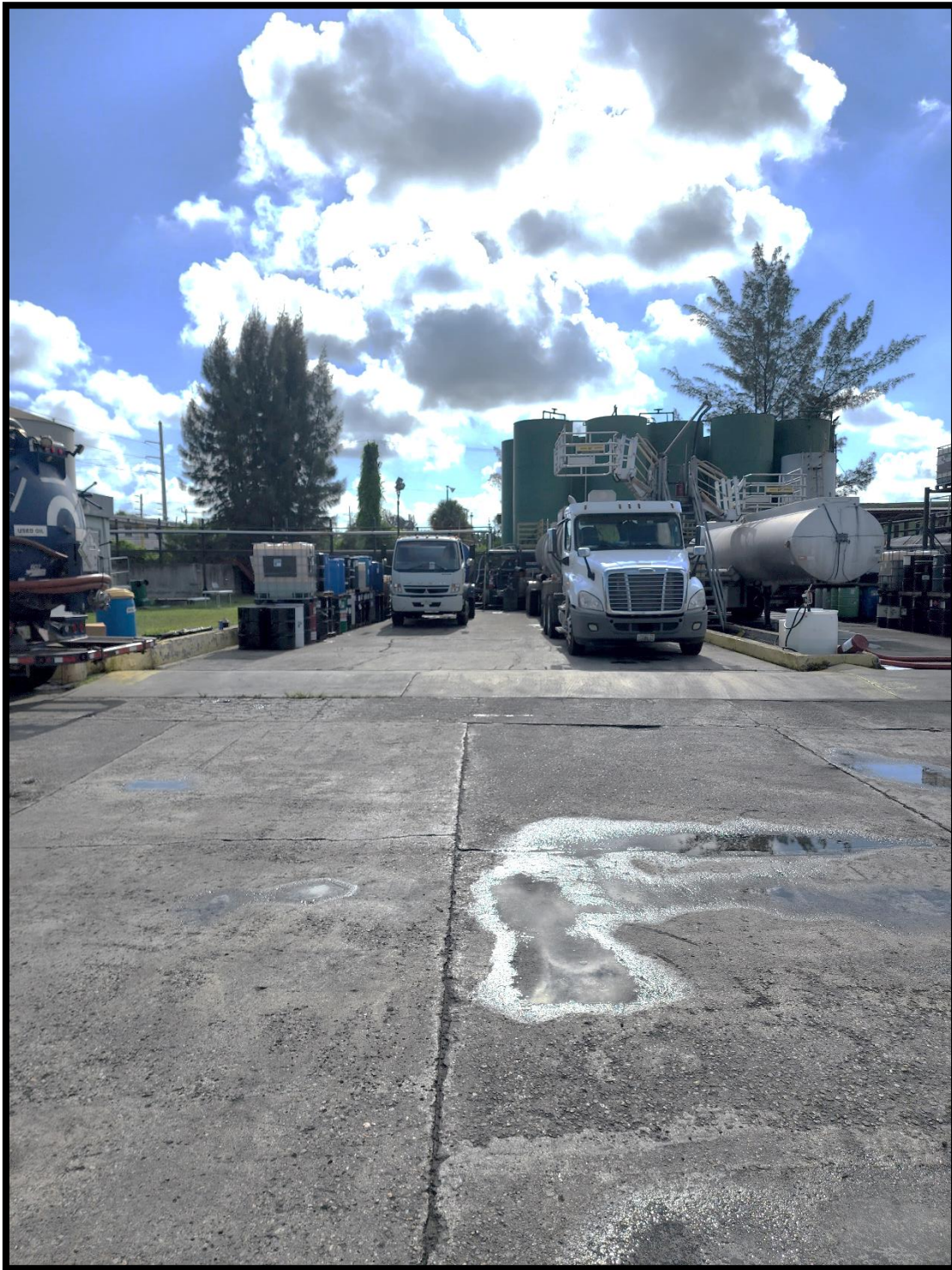
Photo 5: Tanker Unloading Area with Secondary Containment #3 (View from the West)
