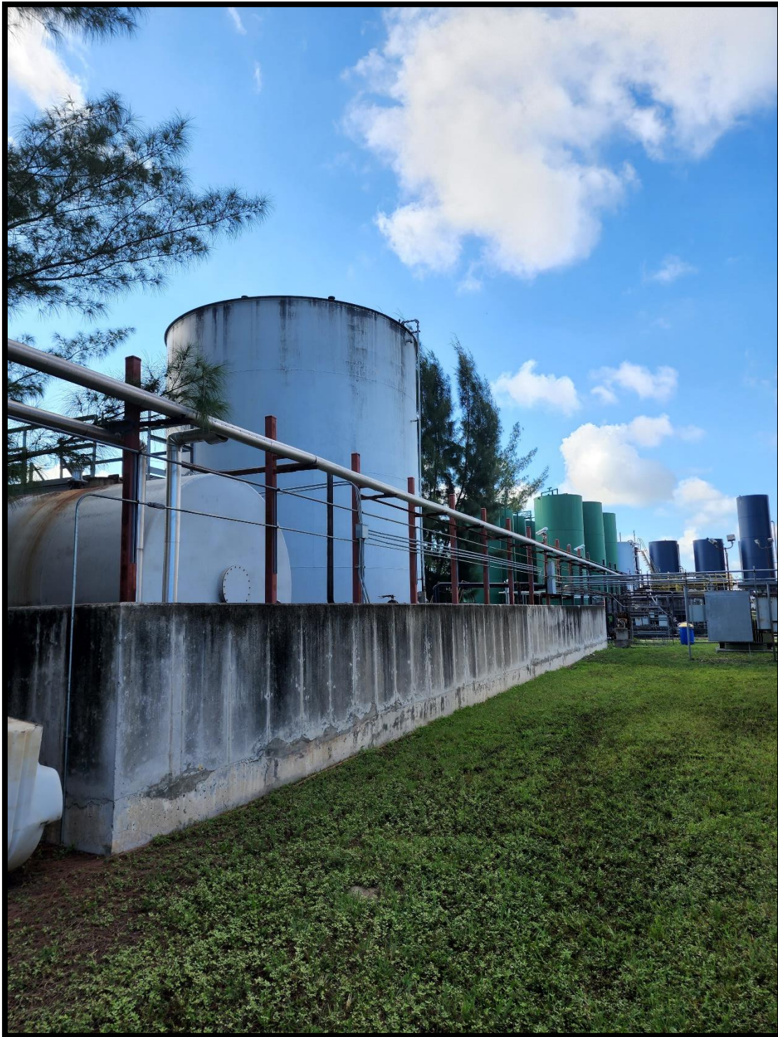
Photo 11: Tank 21/22 (foreground) and Tank 1-18 (background) (View from the North)
