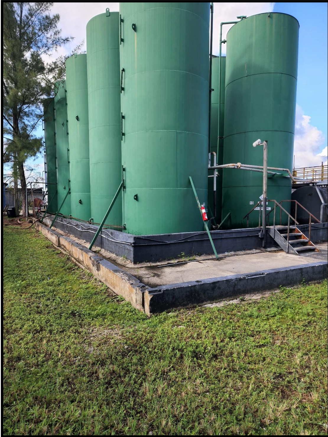
Photo 8: Vertical Aboveground Storage Tanks with Secondary Containment #1 (View from the Northeast)
