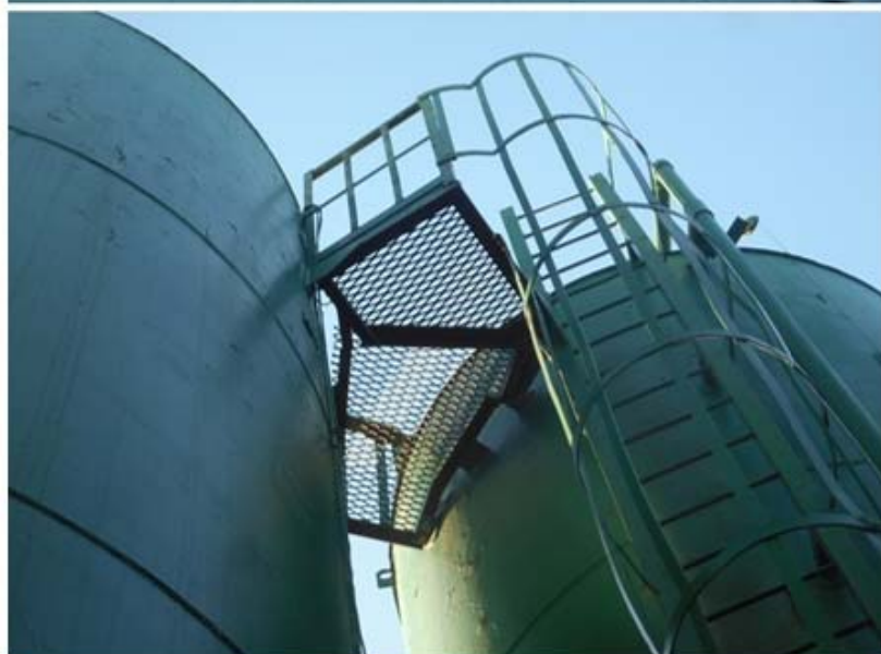
ACCESS FROM ADJACENT TO TANK #16
