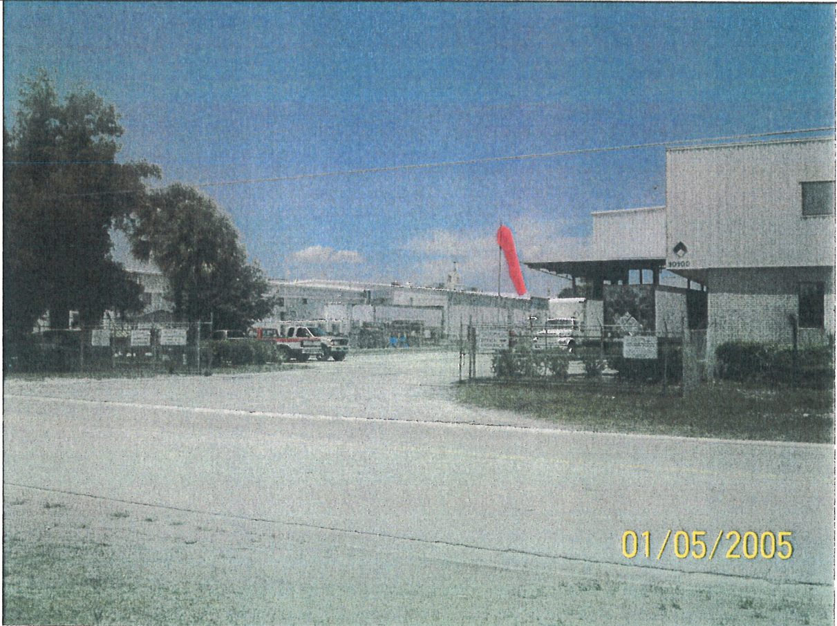
Photo I.B.3.-17: Front of Facility Showing Truck Entrance
