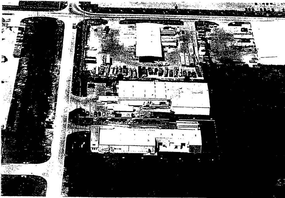
PHOTO I.B. 3-5. FACILITY AERIAL VIEW; TAKEN FROM THE EAST
