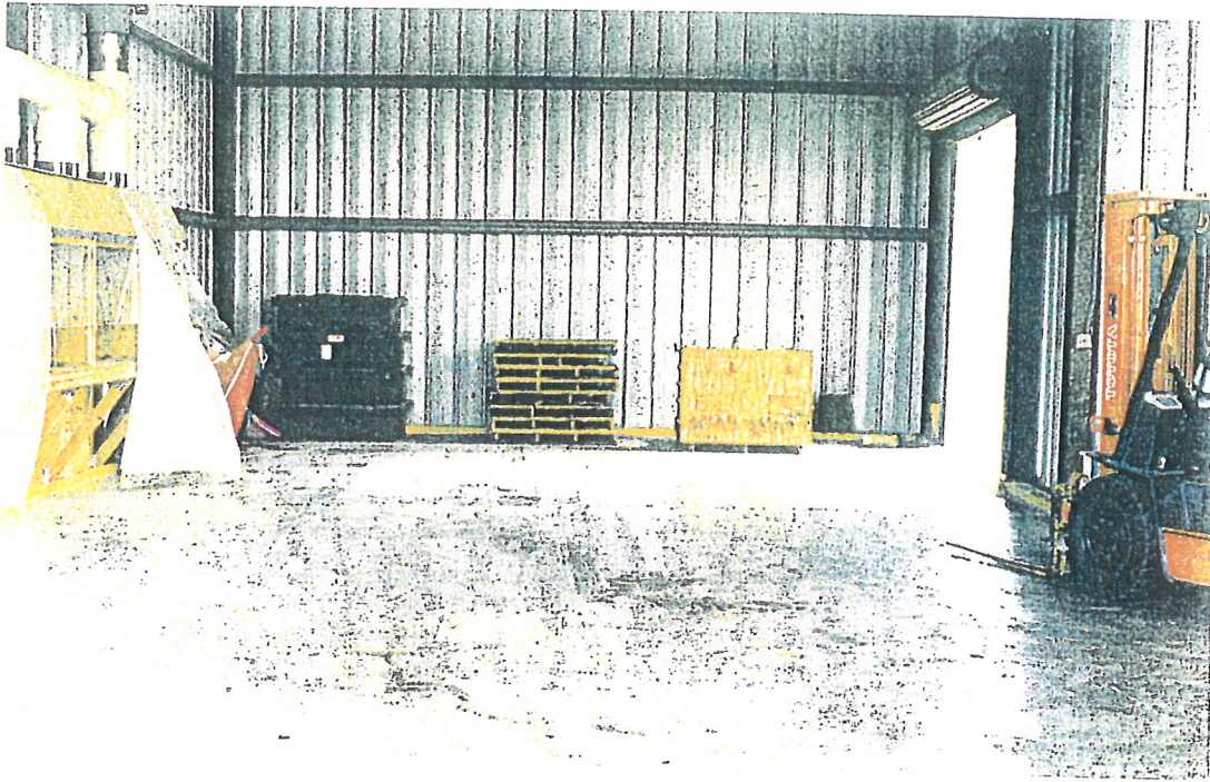
Photo I.B.3.-12 North Building Waste Stabilization/Consolidation Area
