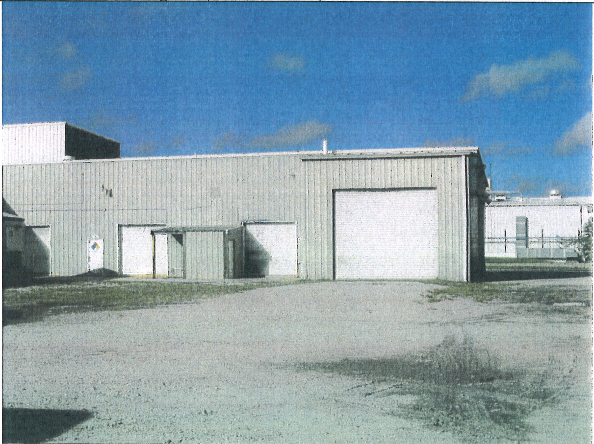
Photo I.B.3.-11: North Building Location for Inside Consolidation/Stabilization Area, View from the East
