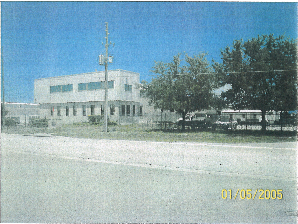
Photo I.B.3.-16: Front of Facility Looking Northwest
