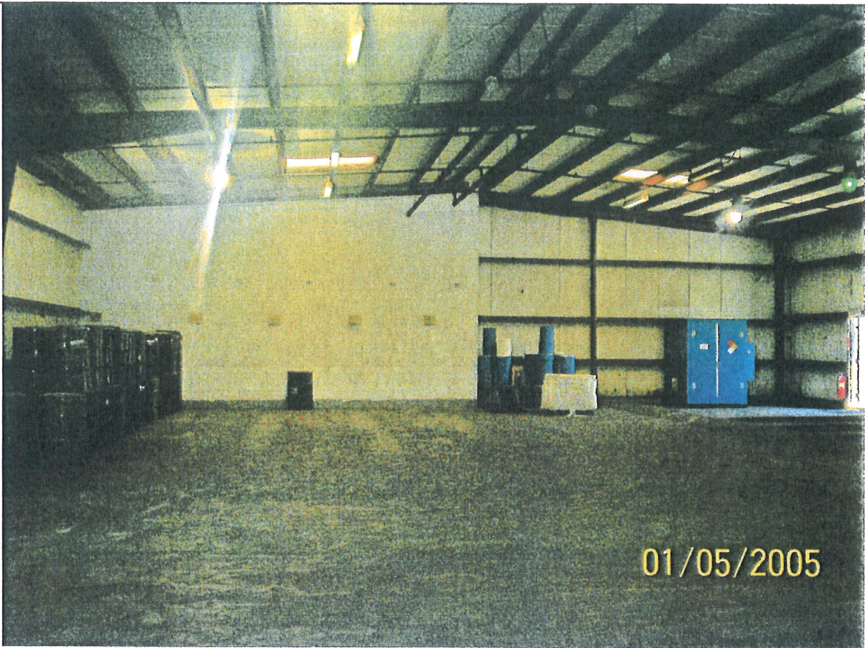
Photo I.B.3.-10: Container Storage Unit, Northwest Area, View From the South
