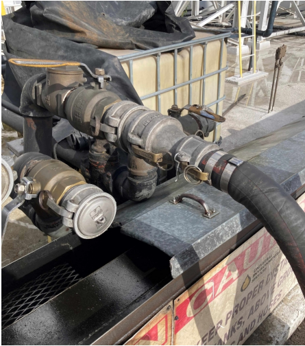
Photo 3 Drain and fill ports
