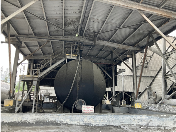
Used Oil holding tanks
