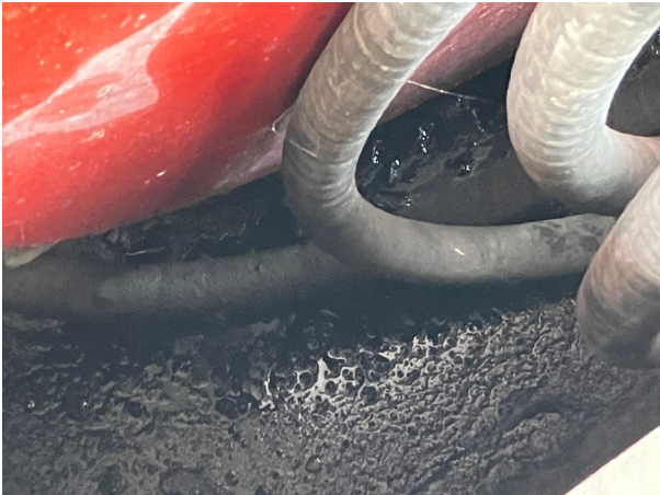
Oil release in secondary containment
