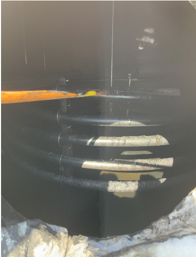
Tank #104 - used oil removed, oily sludge present
