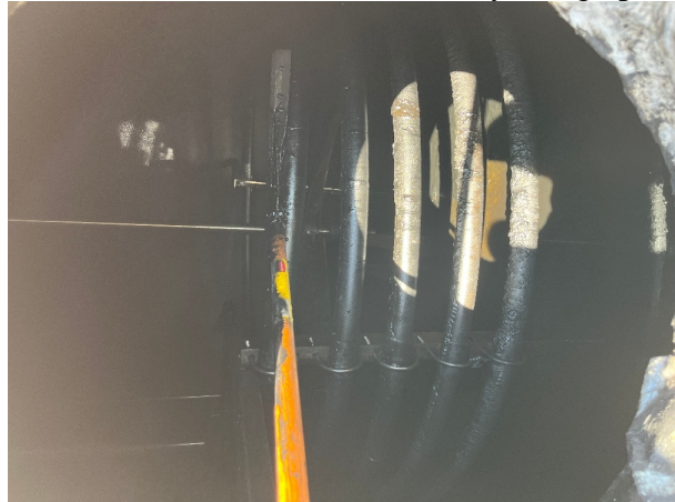
Tank #103 - used oil removed, oily sludge present
