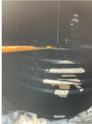
Tank #103 - used oil removed, oily sludge present
