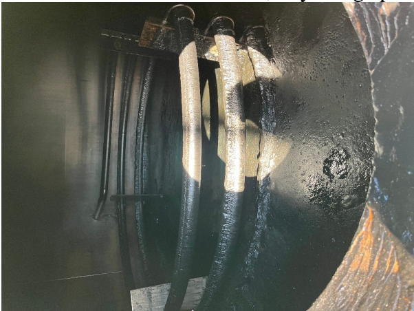
Tank #104 - used oil removed, oily sludge present
