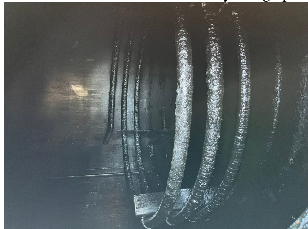
Tank #105 - used oil removed, oily sludge present
