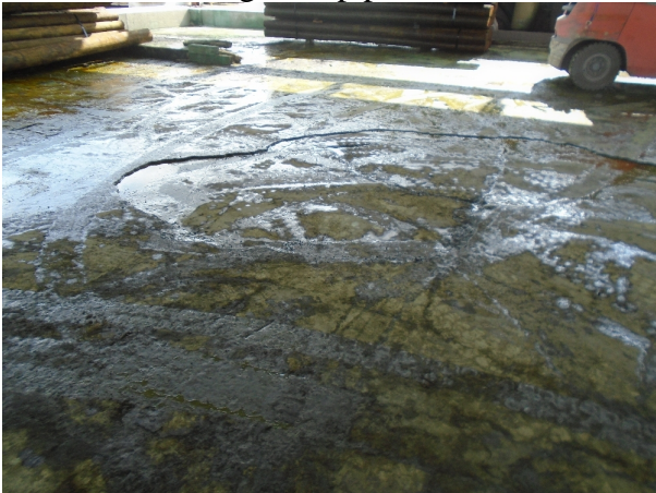
Photo 19 - Damaged drip pad surface and no sealant
