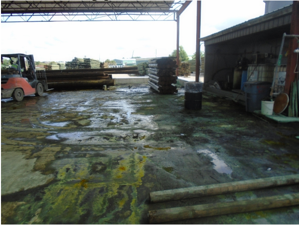
Photo 13 - Damaged drip pad surface and no sealant
