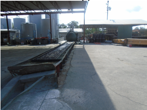
Photo 1 - South end of drip pad
