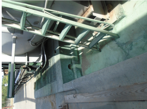
Photo 6 - Cylinder secondary containment sump
