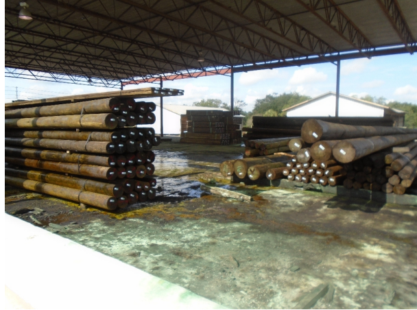
Photo 12 - Damaged drip pad surface and no sealant
