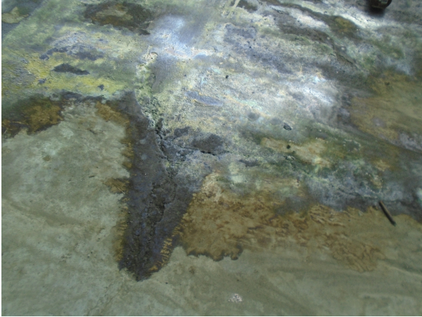
Photo 17 - Damaged drip pad surface and no sealant
