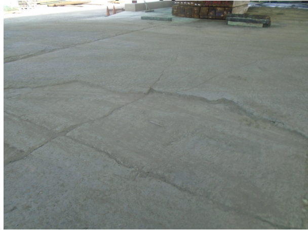
Photo 14 - Damaged drip pad surface and no sealant
