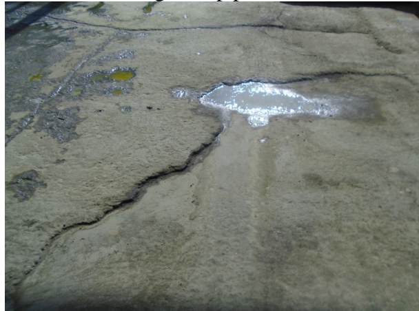
Photo 14 - Damaged drip pad surface and no sealant
