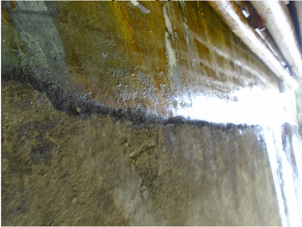
Photo 19 - Damaged drip pad surface and no sealant
