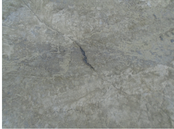
Photo 18 - Damaged drip pad surface
