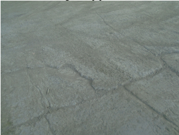
Photo 13 - Damaged drip pad surface and no sealant
