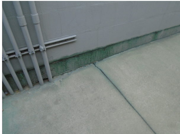
Photo 26 - Hazardous waste release from tank farm 2nd containment
