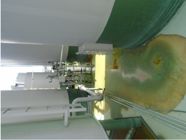
Photo 7 - Leaking cylinder ancillary equipment
