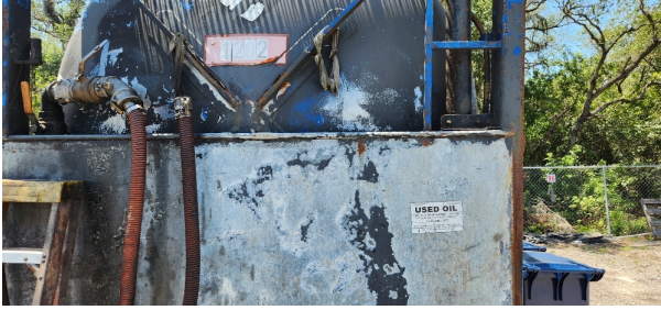
Labeled Used Oil Tank ~6,400 gallons
