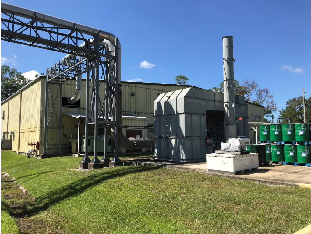
Photo 5. Regenerative Thermal Oxidizer (RTO) (09/2019)
