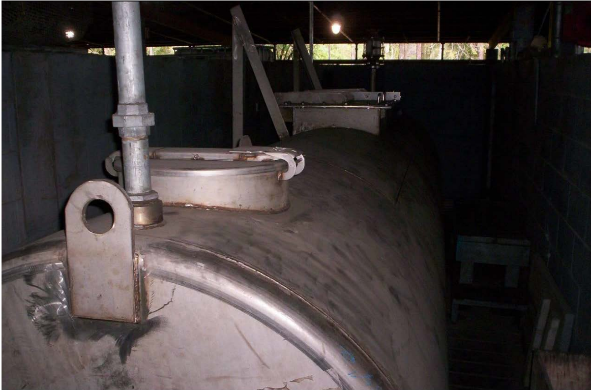
Photo 13. PSB 3,000-Gallon Storage Tank (12/2014)
