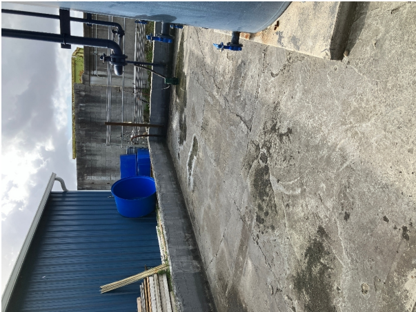
Damaged Secondary Containment
