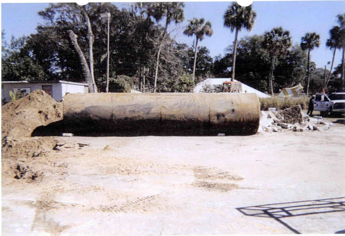
Photograph 3 - View of UST #4 after removal from the excavation.
