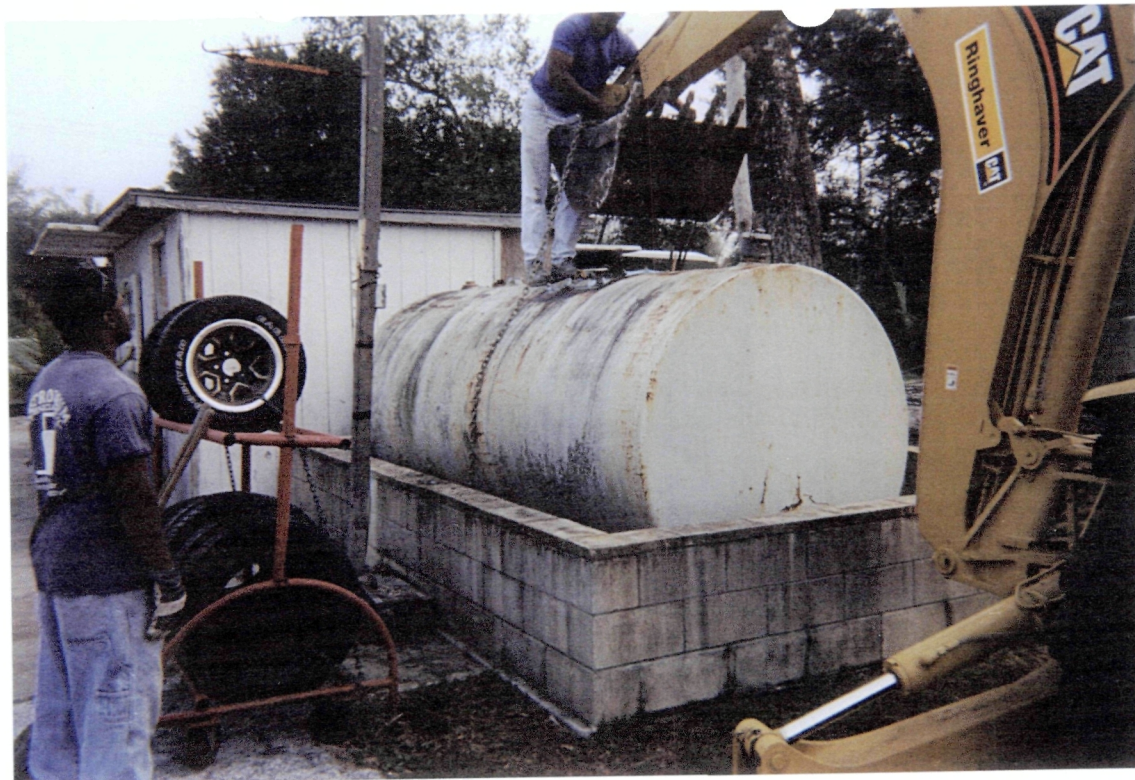
Photograph 5 - View facing north of the diesel AST prior to removal from the secondary containment.
