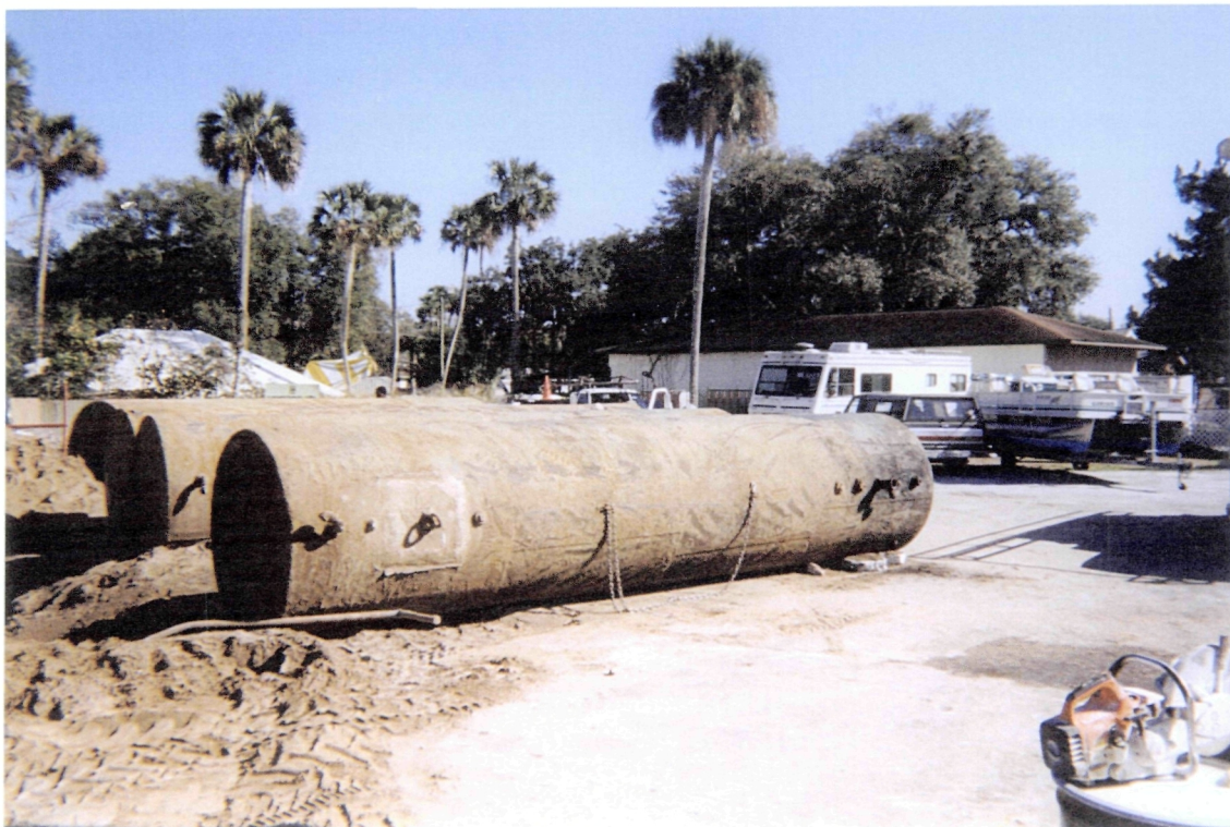
Photograph 4 - View of UST #5 after removal from the excavation.
