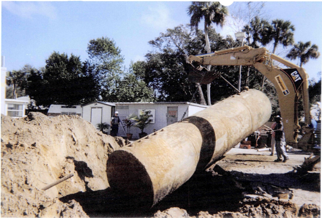
Photograph 1 - View facing east of UST #3 during removal from the excavation.
