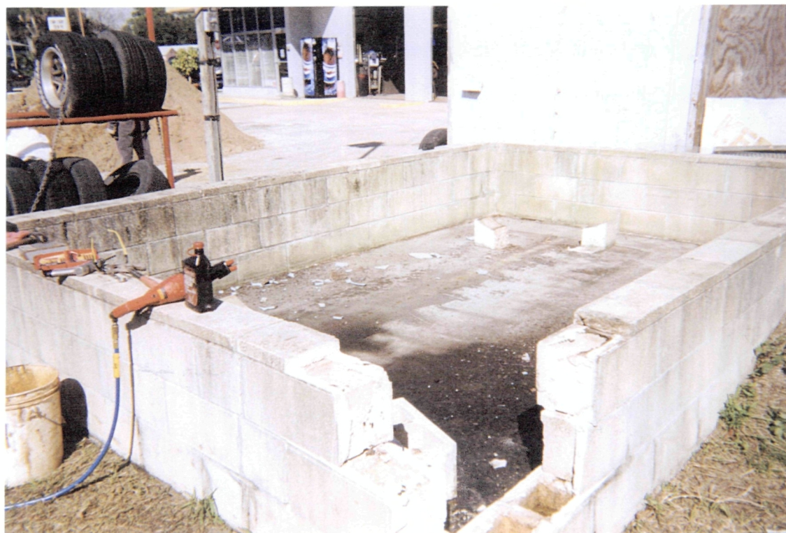
Photograph 6 - View of diesel AST secondary containment after tank removal.
