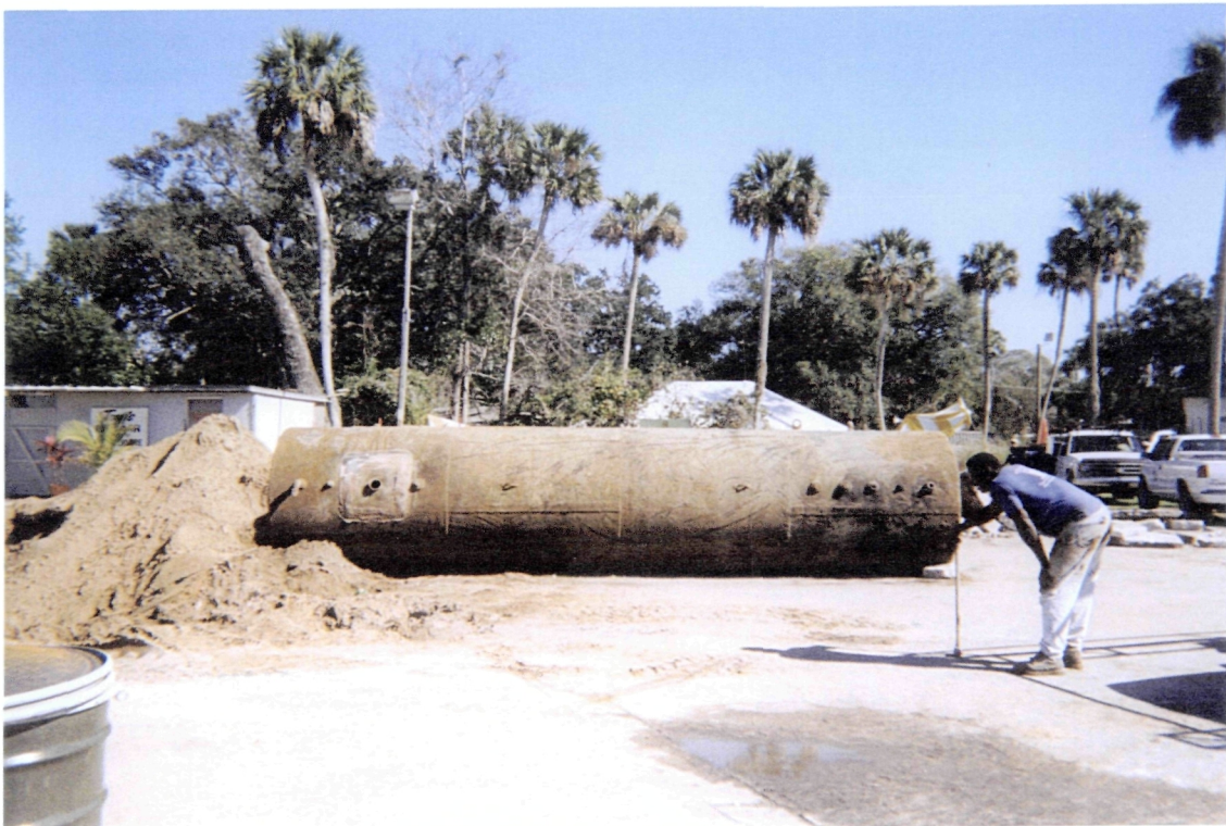
Photograph 2 - View of UST #3 after removal from the excavation.
