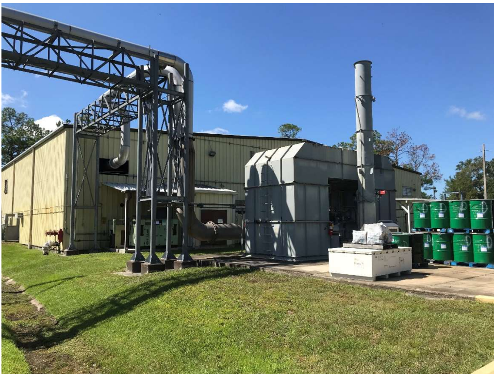
Photo 5. Regenerative Thermal Oxidizer (RTO) (09/2019)
