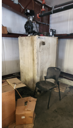
Used Oil Burner Tank
