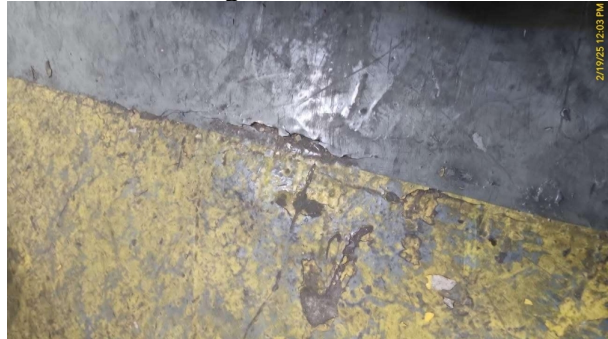
Photo 58 - Damaged floor sealant
