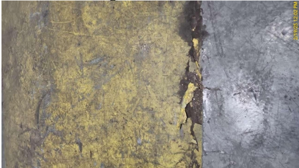
Photo 57 - Damaged floor sealant
