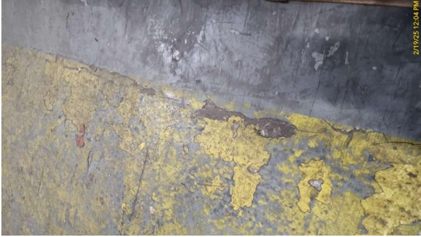
Photo 61 - Damaged floor sealant
