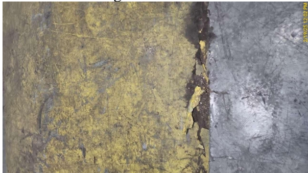
Photo 57 - Damaged floor sealant
