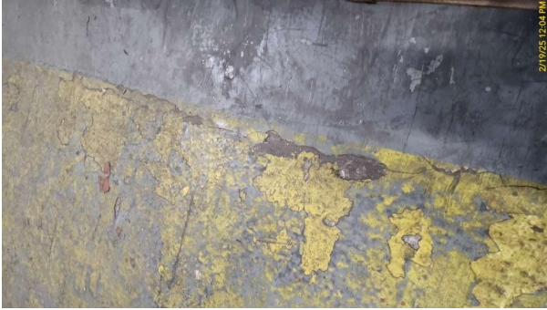
Photo 61 - Damaged floor sealant
