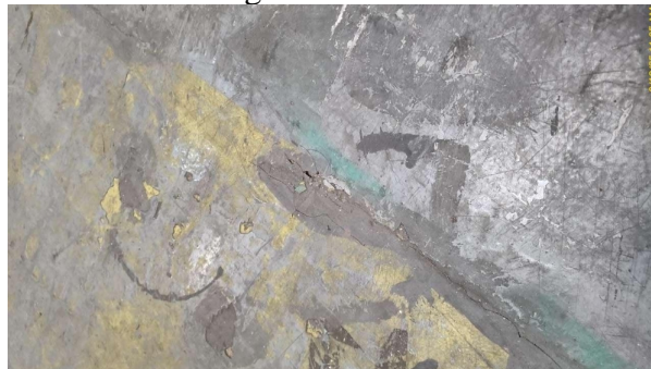
Photo 58 - Damaged floor sealant
