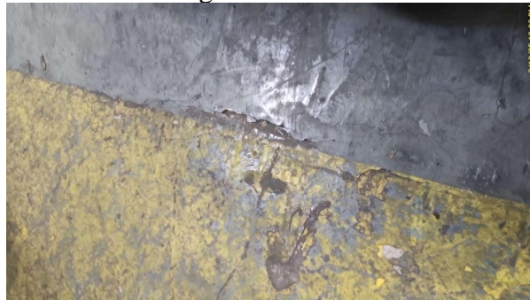
Photo 58 - Damaged floor sealant
