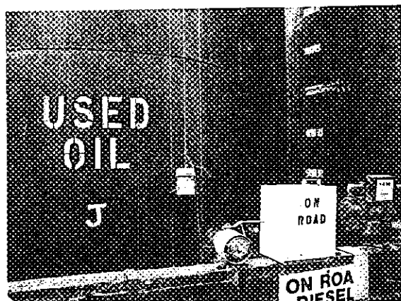
Figure 4. Float indicates tank contains waste
