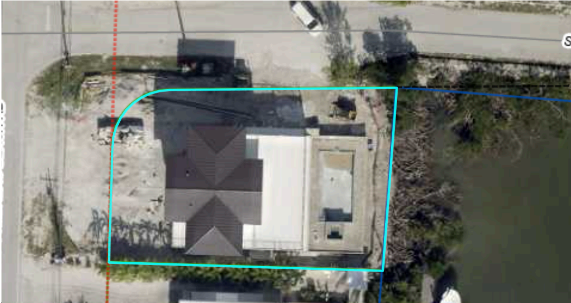
Aerial Imagery – 2023 – Showing Residual Impacts from Hurricane Irma Credit: Monroe County Property Appraiser
