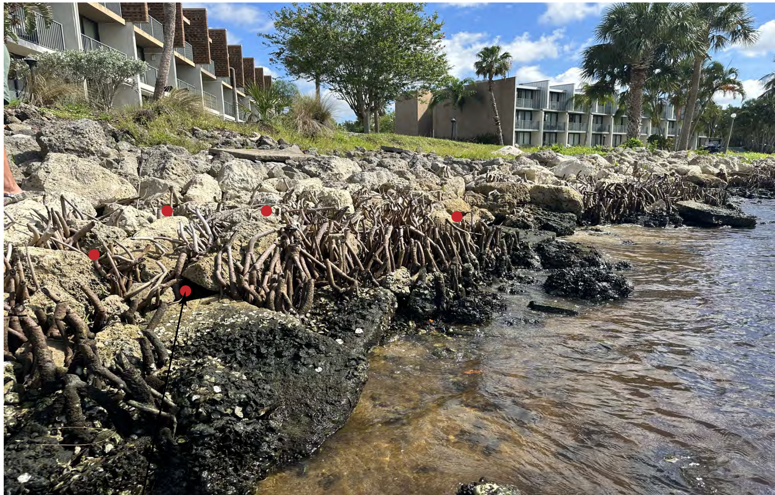
Replanting with mature, 2 ft. tall, Red mangrove seedlings amongst existing riprap. One to one and a half feet on center.
