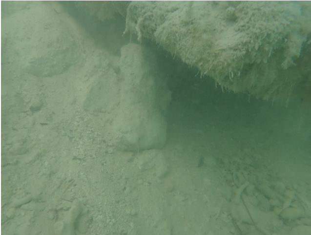
Damage from undercutting
