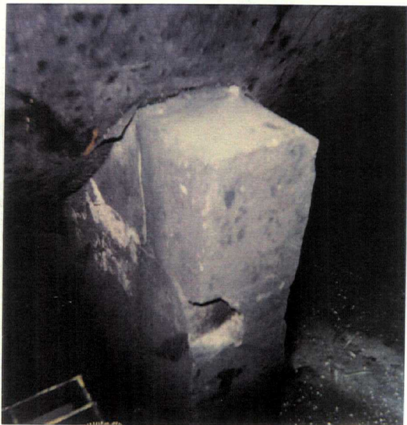
HOWCO 5-15-96 EMR WEST FARM 528624557 TANK #130 WEST MIDDLE SADDLE CRACKING
