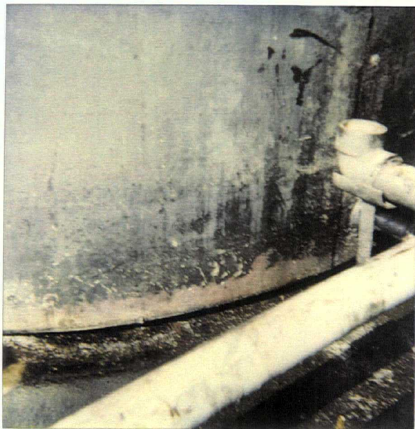
528624557 1-17-96 T120 deformed bottom ER/IS
