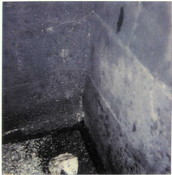
HOWCO 5-15-96 528624557 NORTH LOADING AREA NEAR NW CORNER TANK #100 STEP CRACK & NO MORTAR EMR
