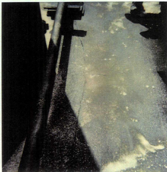
HOWCO 5-15-96 EMR TYPICAL FLOOR 528624557 CRACK, EAST & WEST FARMS
