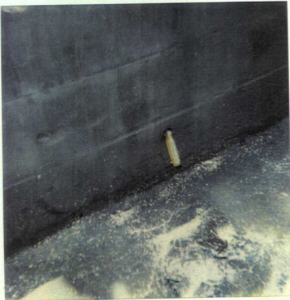
528624557 5-15-96 EMR NORTH LOADING AREA DAMAGED & HOLLOW BLOCK WALL NEAR NE CORNER TANK #100
