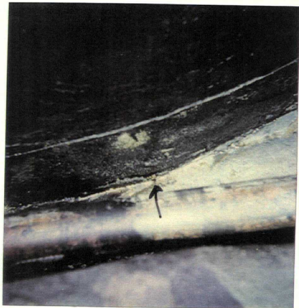
HOWCO 5-15-96 EMR SOUTH LOADING BACK, #173 HOLE AT TANK BASE "7:30 position" 528624557 PHOTO # 6
